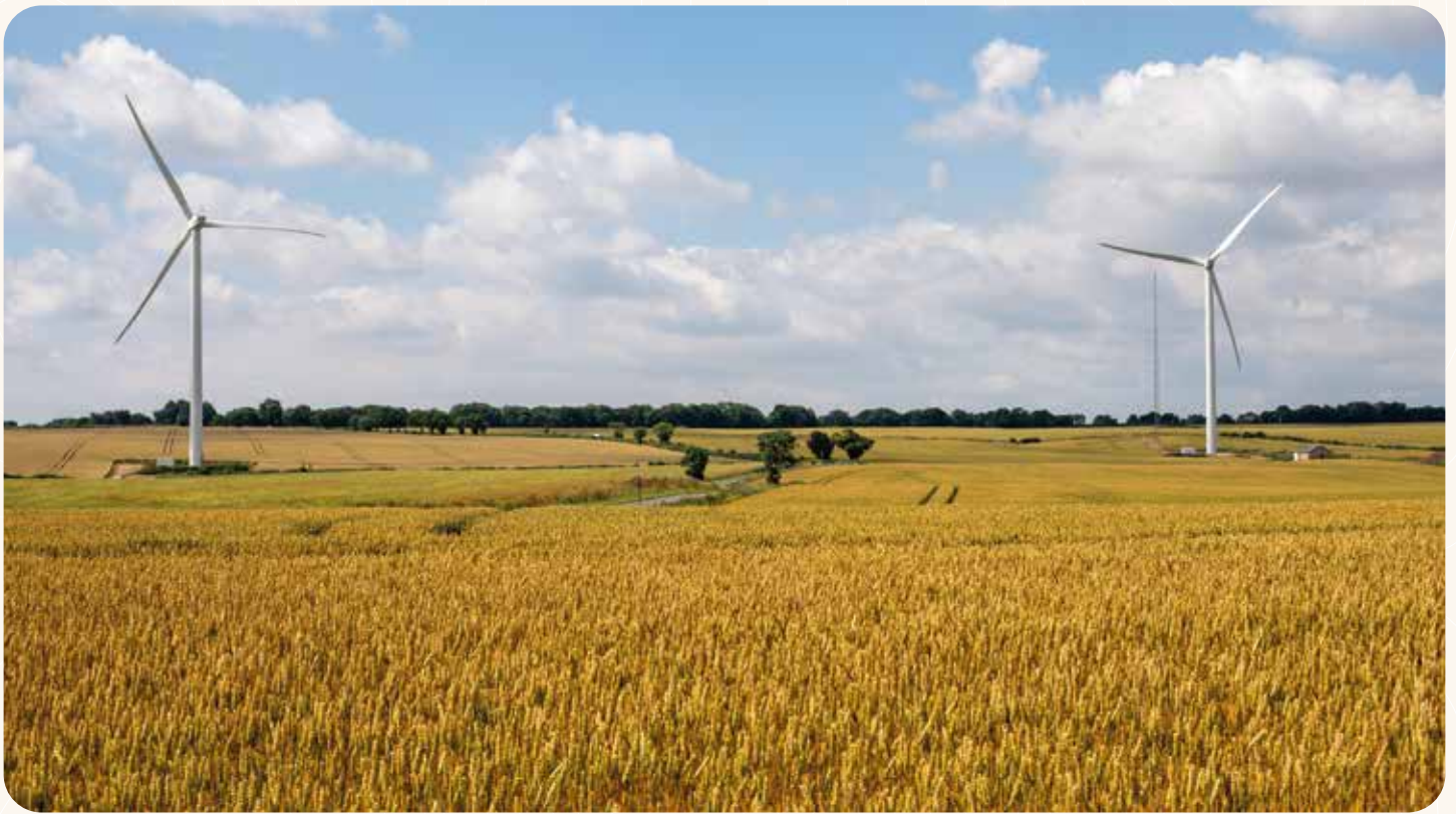
Marr Wind Farm near Doncaster
